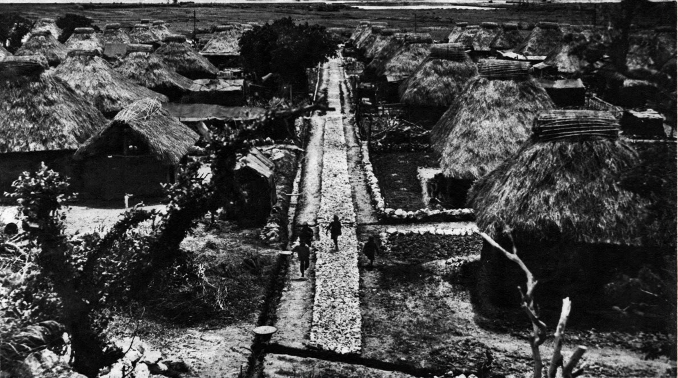
Typical thatched-hut village of prefabricated houses overlooking Buckner Bay. The American housing program has produced prefabricated frames for 40,000 huts, enough to get a half-million Okinawans out of the caves and hills where they had taken refuge. The military government's goal is 100,000 of these new homes
